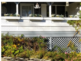
Lattice (below porch)
