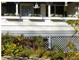
Lattice (below porch)
